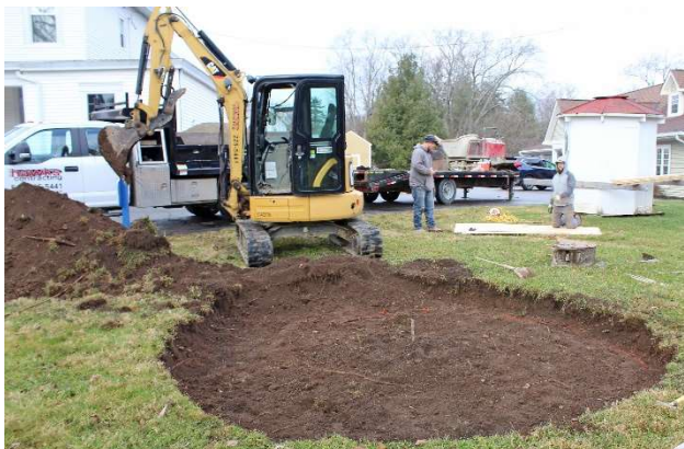
First workers dig the hole
