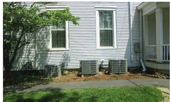
Bonaventure after bushes were removed
